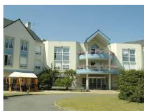
RESIDENCE ANDRE ROCHEFORT
